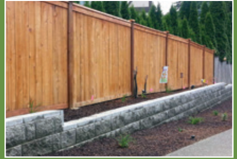
Grades and Retaining Wall Examples
