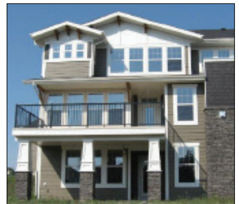
Rear Facade Examples
